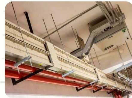
Installation of busduct system Paseo San Francisco
